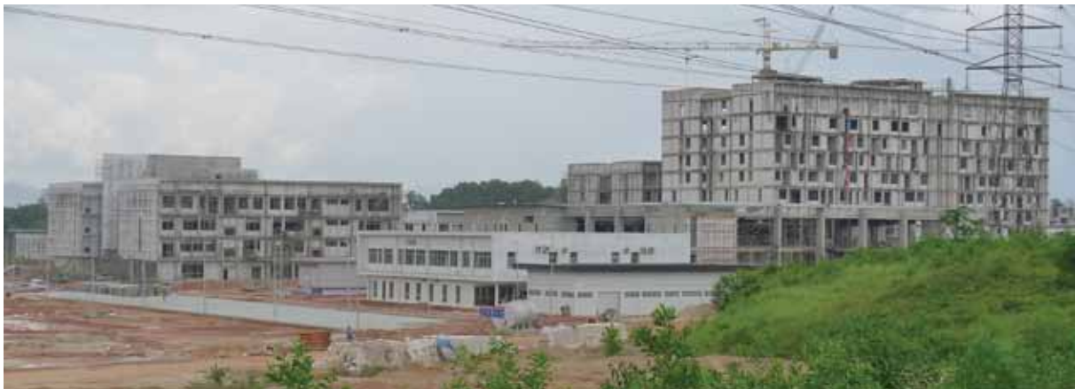
UiTM Campus, Seremban 3, Progress Status At 2 November 2011
